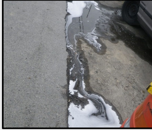
Suds often enter storm water systems as a result of improperly connected car washes or washing machines. Sude can aslo be the result of improper vehicle washing practices.
